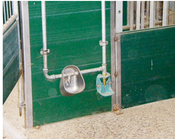
To ensure a good water supply for the weaned piglets, there must be enough drinking bowls available at a suitable height.
